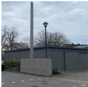
Picture on left showing a single AWC8063 Cabinet to the left of the AWC8062 Pole Surround Enclosure and two AWC8061 Cabinets positioned to the right of the Pole Surround Enclosure.
