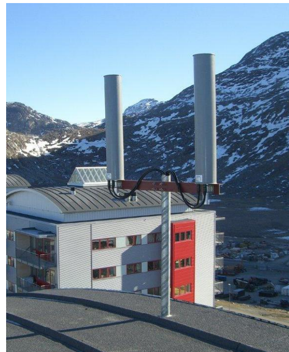
Figure 1 – Typical modern roof-top antenna system
