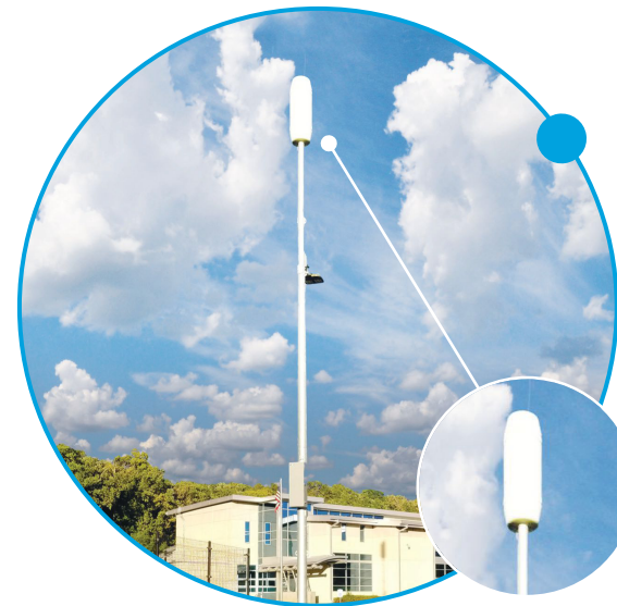
CAN DEPLOYMENT, KANSAS CITY, USA
