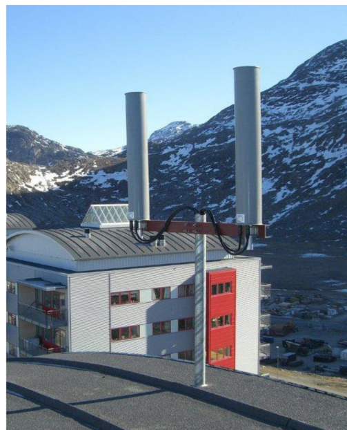
Figure 1 – Typical modern roof-top antenna system
